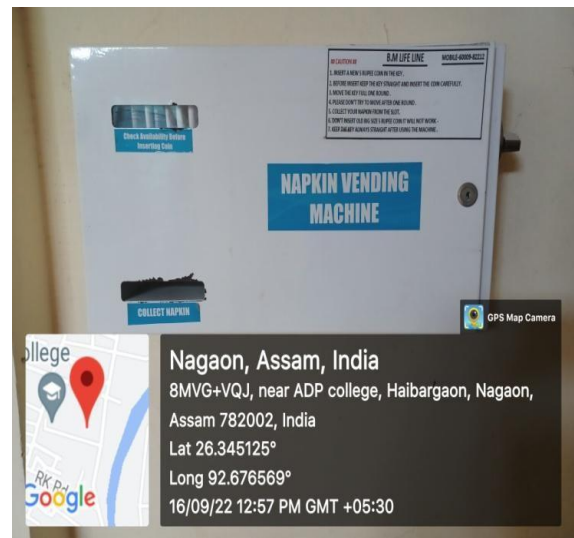
Installation of Sanitary Vending
